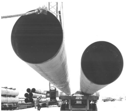
Alyeska Project 48 inch diameter/80 foot length pipe haul by Alaska Railroad from Valdez
