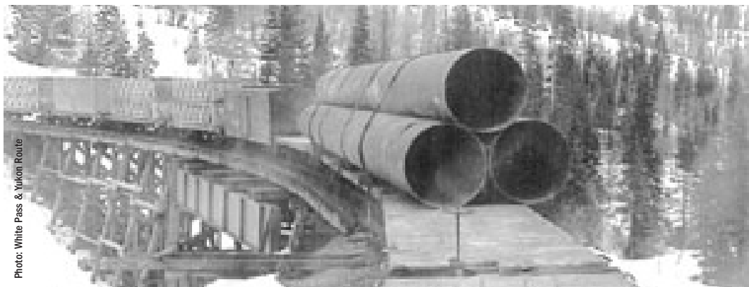
Foothills Project 56 inch diameter/80 foot length pipe haul test by White Pass & Yukon Route
