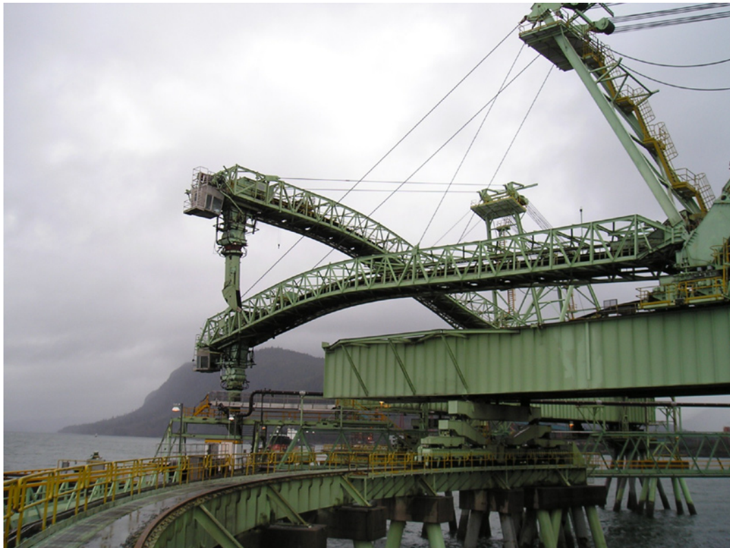
Ridley Island Coal Terminal, Prince Rupert, B.C.
